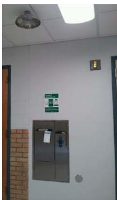
The *eyewash unit* is activated by pulling open the door. The water will begin to flow automatically from the nozzles so you can flush your eyes. This water can also be used to wash exposure to hands. Be sure to hold your eyelids open and flush eyes for at least 15 minutes.
