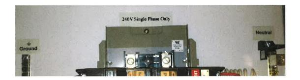
When connecting the components to the system make sure power is completely shut off prior to making the connections. Take care to note the plug's orientation as they only go in one way. Do not force the plug as it will cause damage. All connectors are twist lock.
